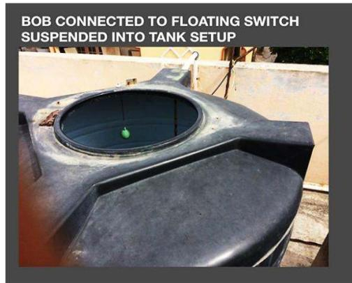
Figure 4. Bob connected floating switch suspended into water tank
