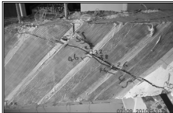
Fig. 11: Shear failure of Beam 2-4 at load 380.74kN (shear force 124.69kN)
