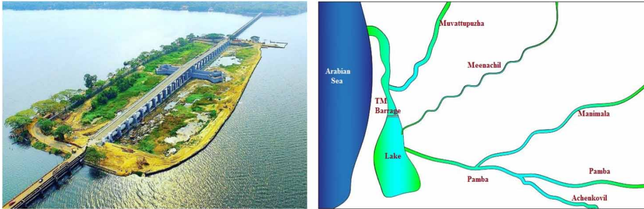
Figure 5 | (a) Bird's eye view of Thanneermukkom barrage; (b) location of barrage across Vembanadu Lake.
