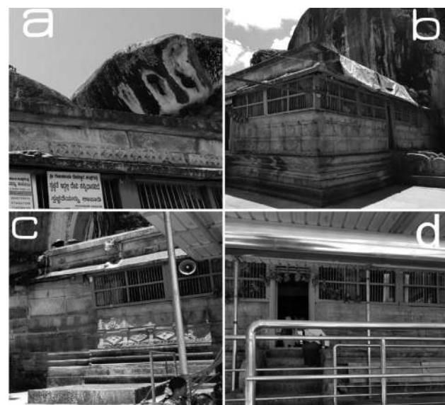
Figure 2: Renukadevi Temple, Karnataka, India: a) top view of the temple, b, c) side view, d) entrance to the temple
