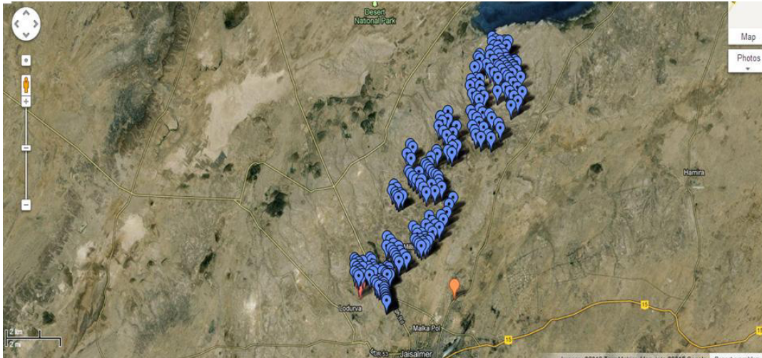
Fig. 6. Cluster of Wind Turbines at the Jaisalmer Wind Park as of December 2012
