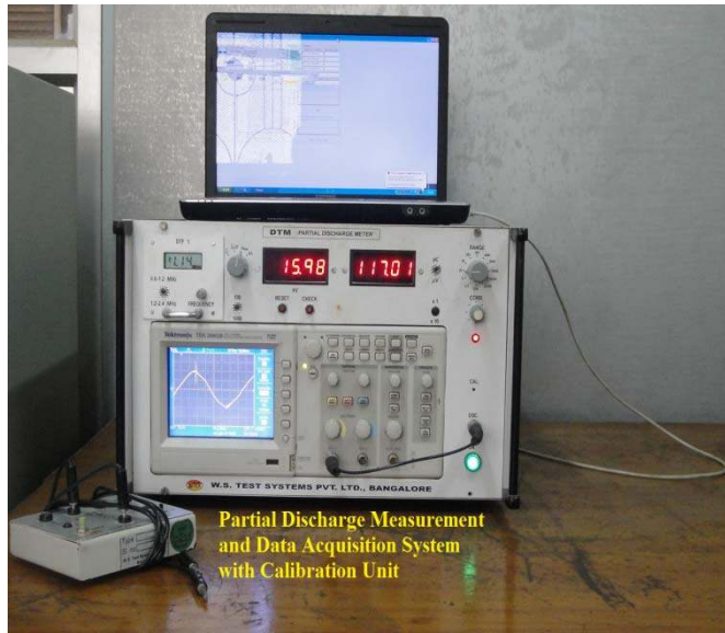
Figure 4. Partial Discharge Measurement and Data Acquisition System
