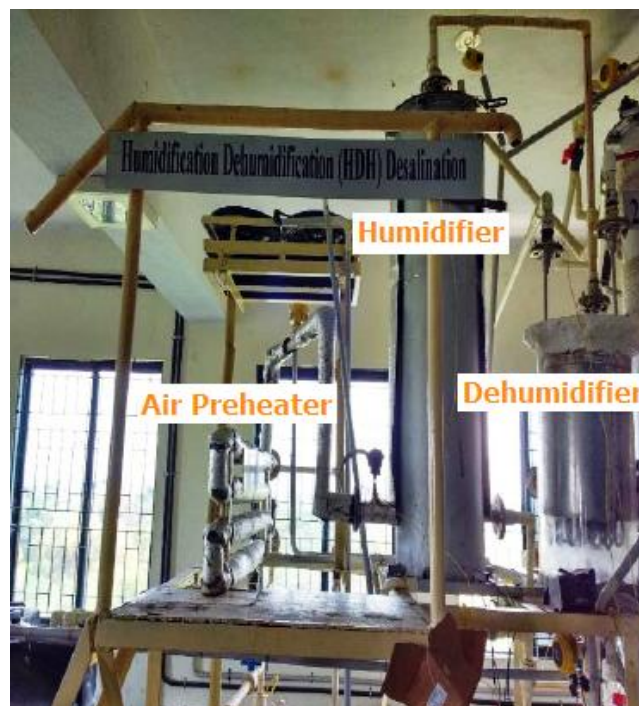
Figure 2. Photograph of solar humidification dehumidification desalination plant.
