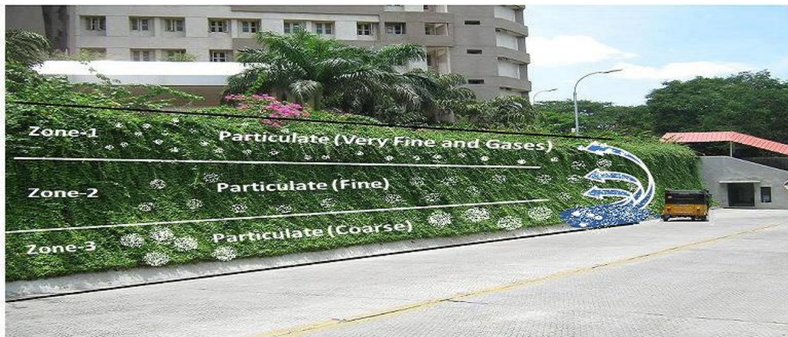
Figure 14: Schematic diagram - dispersion of particulates and gases throughout the height profile of the subway wall.
