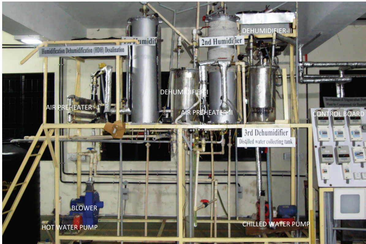
Fig. 2. Experimental setup of two stage HDH desalination and cooling plant.
