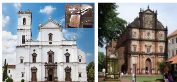
FIGURE 6. Damaged roof and gables due to lightning strikes in Se Cathedral and Basilica of Bom Churches at Goa during 2015 and 2016 respectively
