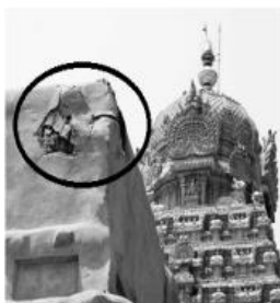
FIGURE 2. Brihadishvara Temple – Lightning strike chipped-off mortar in precincts adjacent to main tower (Sri Vimana) in 2011
