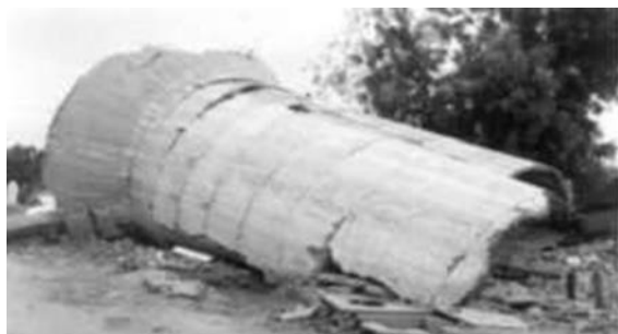
(a) Collapsed circular shaft
