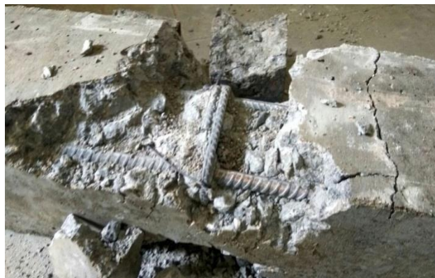
Figure 12. Non- corroded reinforced bars after strength test
