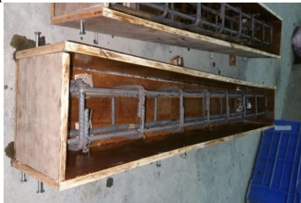
Figure 4. Reinforcement cage inside plywood moulds
